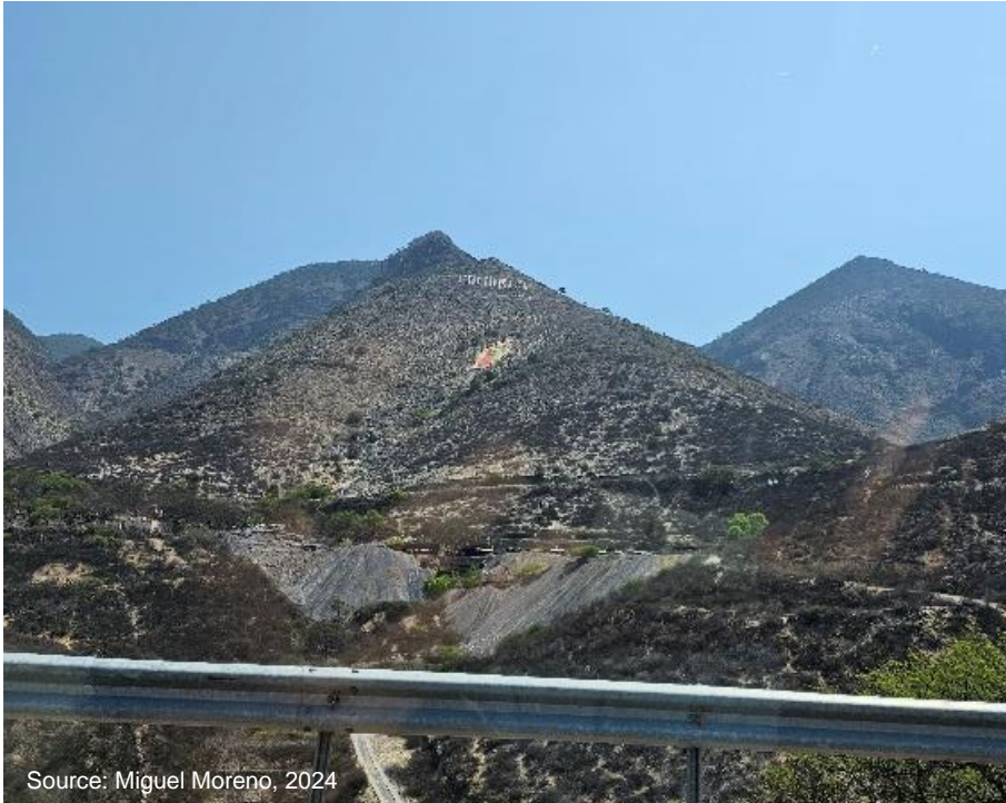
Figure 7. Mine of Camargo seen from the Federal Highway
